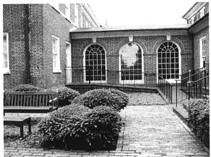
Figure 2: Albemarle County Court House. Ramp entrance. Records Room is on the second floor on the left in the photo. Photograph courtesy of Patricia Lukas, 2016.
